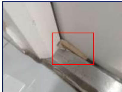
Inserting and blocking emergency exit ladders
